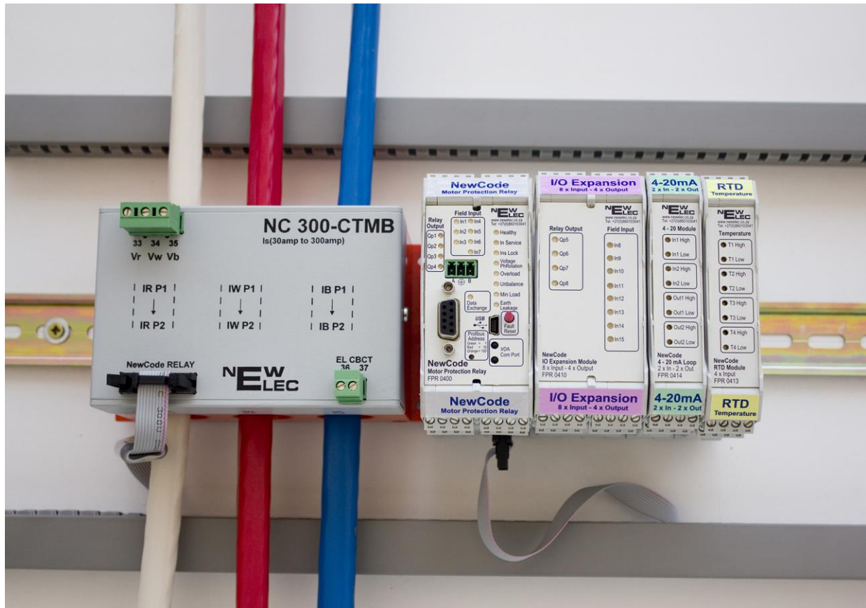
Figure 1: The picture of the NewCode relay, with I/O Expansion, 4-20 mA loop and RTD Modules, is shown.
